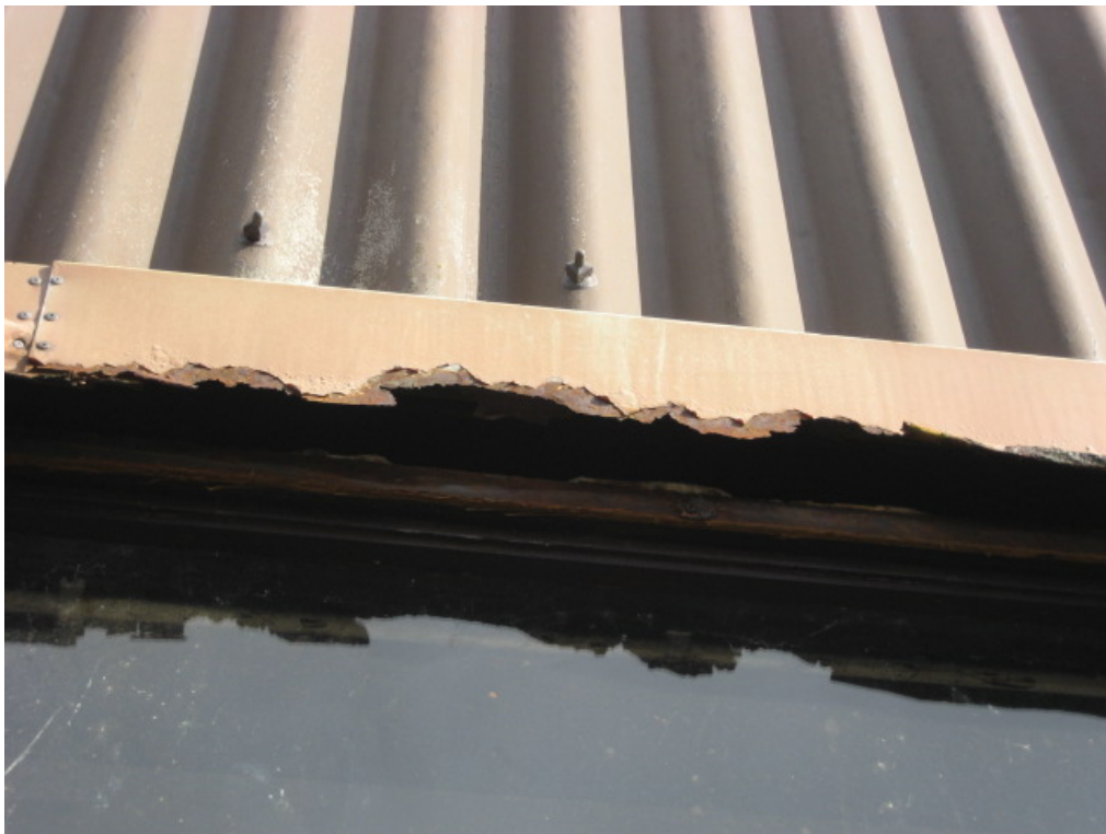
13. Example of spalling
