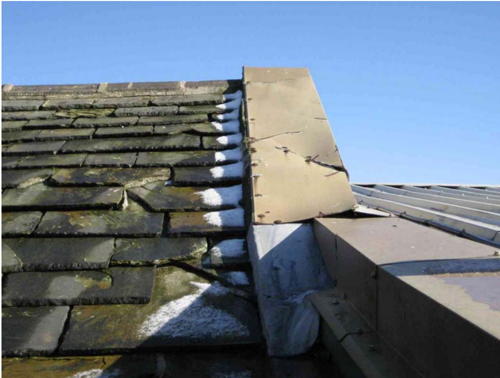
3. Example of decay to stone roof coverings
