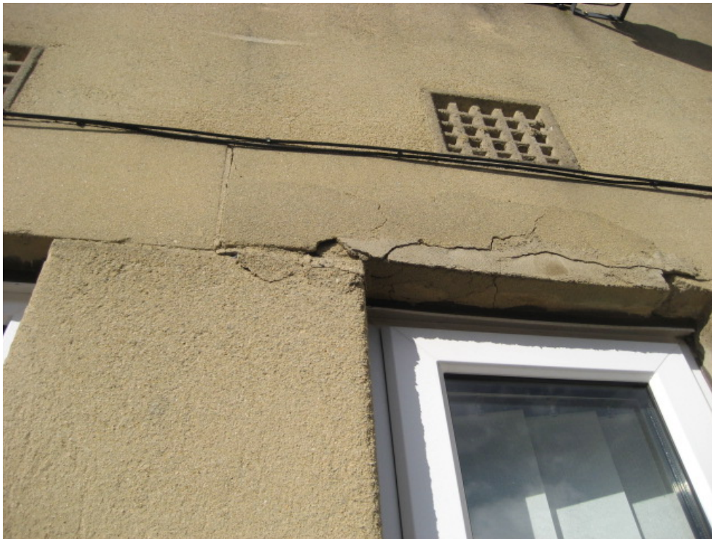
13. Example of spalling
