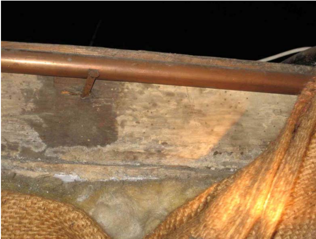
25. Evidence of wood boring beetle attack to building 13
