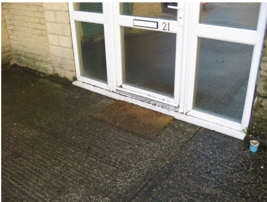
8. Further example of entrance
