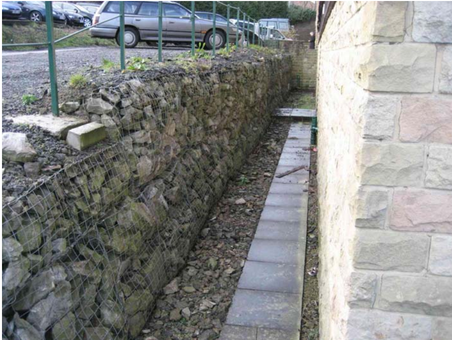
11. Access path to rear building 3
