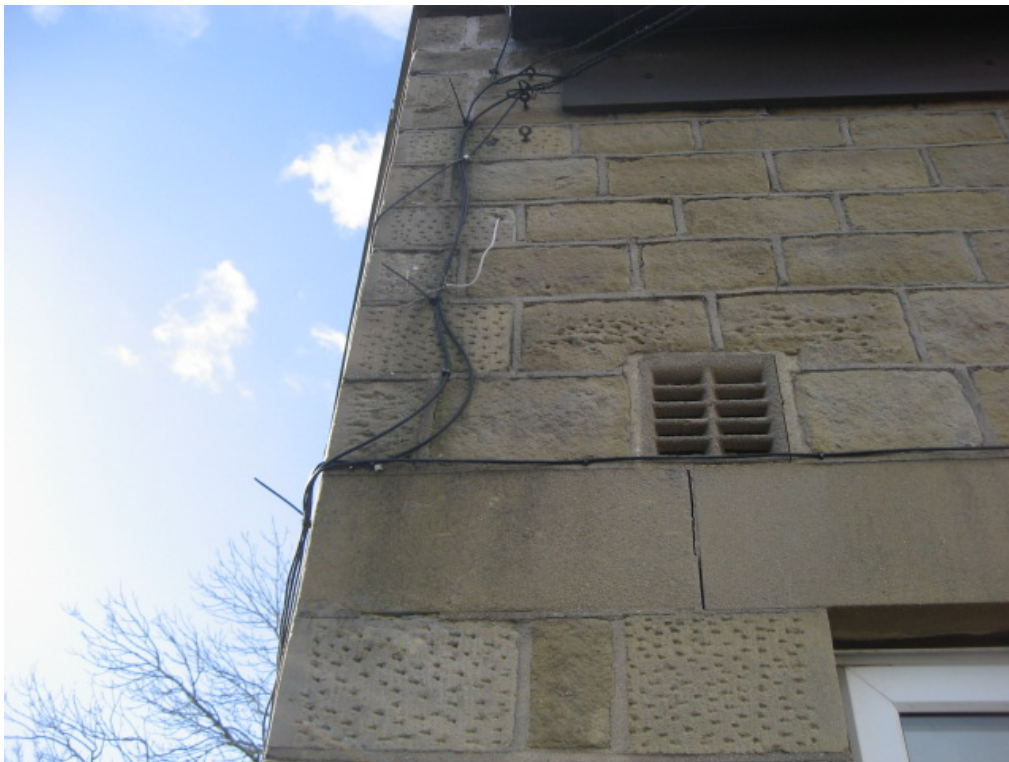
11. Example of cracking
