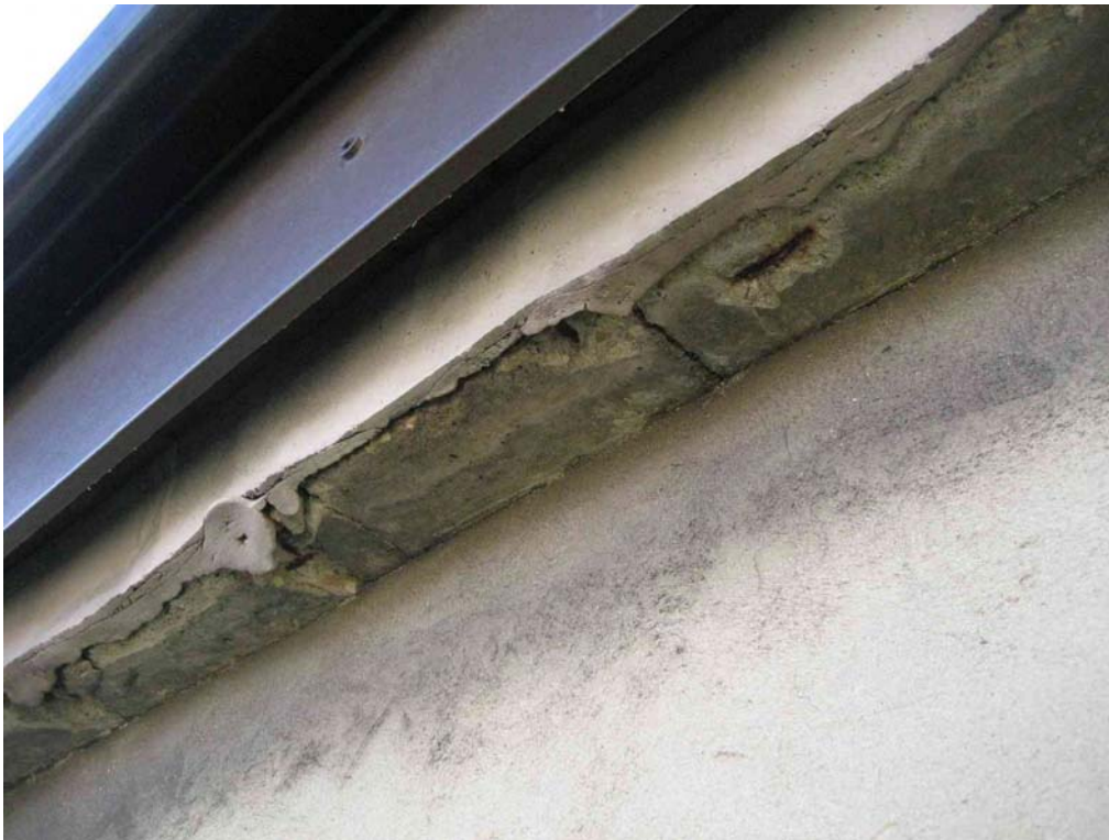
9. Spalling and corrosion to exposed pre-cast concrete units
