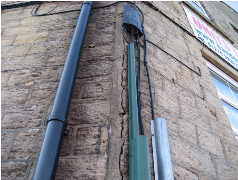
17. Example of cracking
