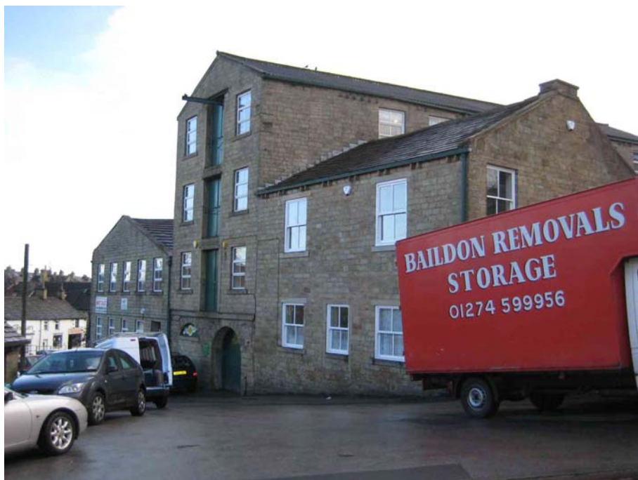
2. View showing slope
