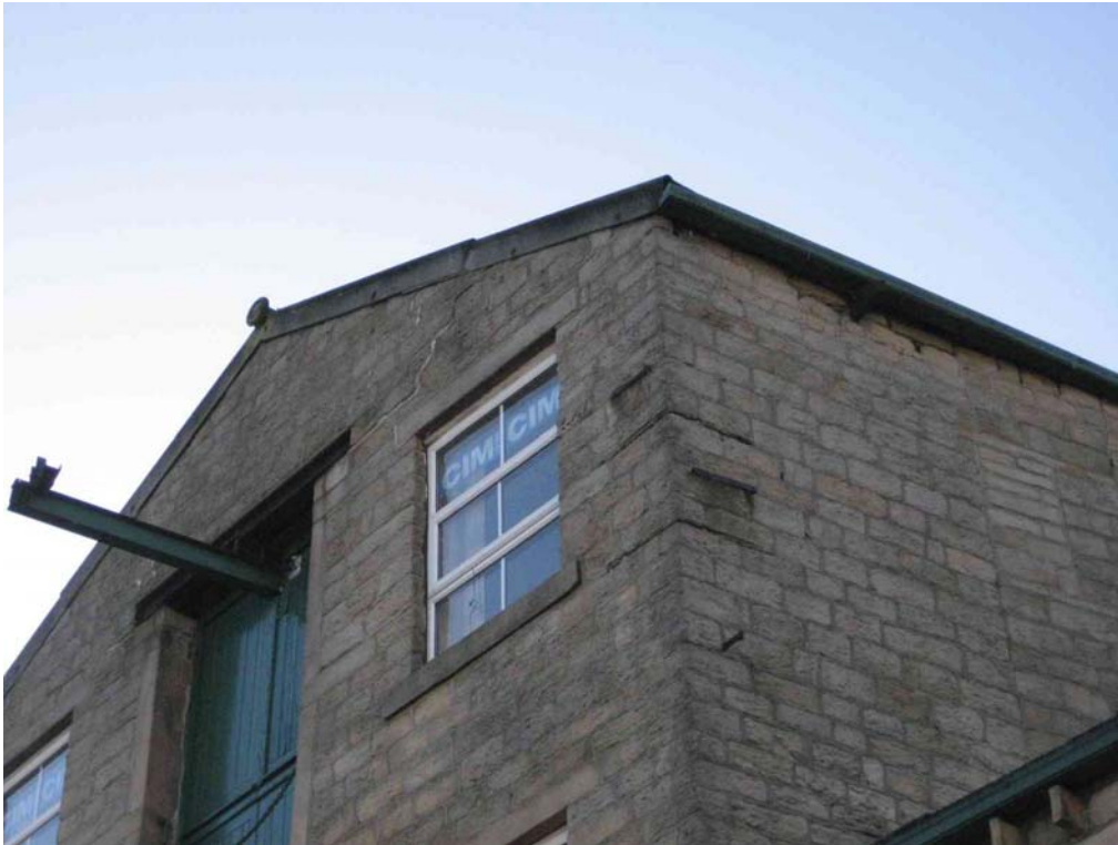
19. Cracking to building 12
