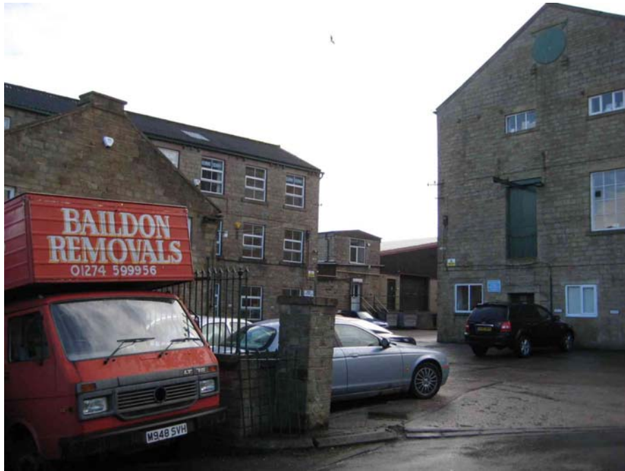
1. Access to main car park
