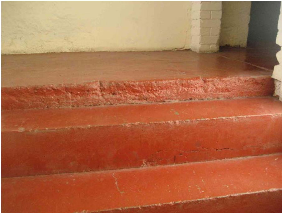
15. Shallow step to stairs to building 1
