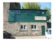
The left side elevation to Block C is cement rendered with stone quoin detailing provided to the corners of the elevations and door openings.
