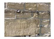
Vertical stepped cracking was noted in 3 nr. locations to the South, East elevation of Block B1. As illustrated in the adjacent photographs the extent of the stepped cracking is Circa. 500mm length and 2mm in width. The extent of cracking is not considered to be significant. We recommend that this is repointed to prevent water ingress and further disrepair. The cracking to this elevation appears to be historic.
