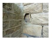
Multiple hairline cracks were noted to the cement based render associated with the South, East elevation of Block C. To prevent water ingress to the fabric of the building all failed areas of render should be hacked off and renewed.
