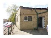
The majority of the original single glazed, timber framed windows have been replaced with modern PVCu double glazed units across all buildings. A single glazed timber framed window remains to the right side elevation of Block B serving the stairwell. Similar to the windows, the majority of the original timber doors have been replaced with PVCu doors. Stepped thresholds are provided to all but two ground level door openings across the site.
