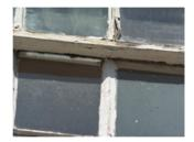
All of the double glazed PVCu windows were generally in fair condition. Three double glazed units have failed with condensation evident. Note trickle vents are not provided to the majority of the windows. To aid background ventilation and reduce humidity levels to the internal aspects of the buildings trickle vents should be installed.
