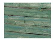
The pointing and the stonework to the North, East elevation of Block C is generally heavily weathered. A number of individual stones are loose and dislodged. We recommend that individual stone repairs are undertaken. Where needed any replacement stone should match the existing in durability and texture to prevent accelerated erosion to the surrounding stonework. Any repointing works undertaken should be completed using a lime based mortar
