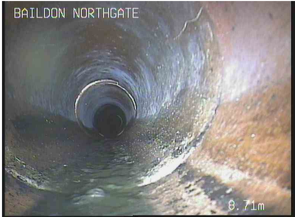
FMH4X_c9c2f2c7-15d8-4bd2-8e2d-85815f63d5a1_20190426_132440_823.jpg, 00:02:02, 8.71m Crack, longitudinal at joint at 02 o'clock
