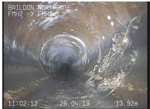
FMH2X_3c1a41a3-a071-49c4-a04a-8a790094ce7b_20190426_120217_308.jpg, 00:04:05, 13.92m Roots, tap
